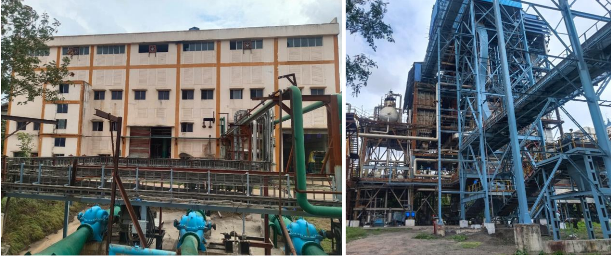
Photographs showing the project site
